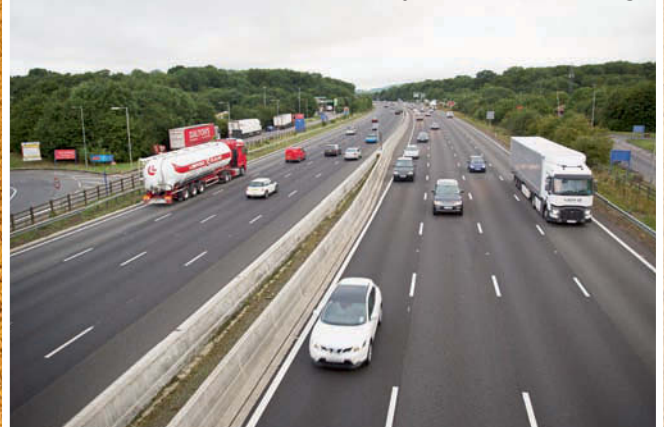
M25 smart motorway with all lane running
